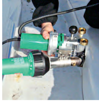
The TRIAC DRIVE PID even allows horizontal welding.
