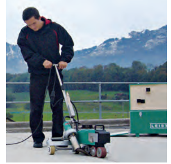
The new VARIMAT V2 in use. Hoisted onto the roof in the practical transport box.
