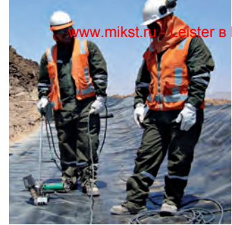
TWINNY S with combiwedge at work at a mining site in South America.
