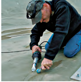
Welding of the connectors with TRIAC PID and push-fit wide slot nozzle.
