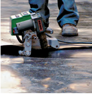
TWINNY T with combiwedge, welding a HD-PE sealing sheeting.
