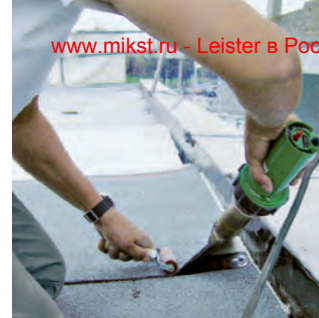
Welding of bitumen sheeting using the powerful ELECTRON with a wide slot nozzle.
