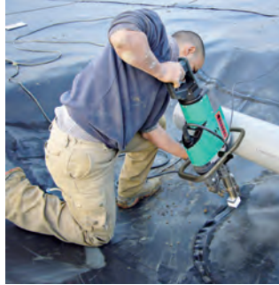
WELDPLAST S6 undertaking assembly applications on a landfill site.
