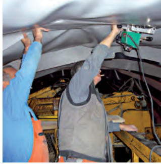
Comet operating in the tunnel
